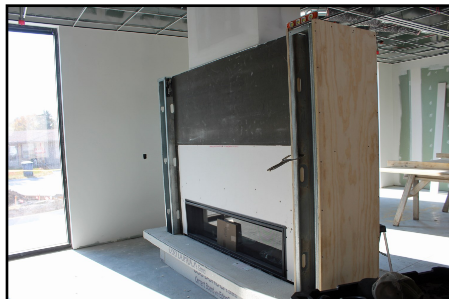
The new fireplace (work in progress) courtesy of Jim and Sharon Crouse.
